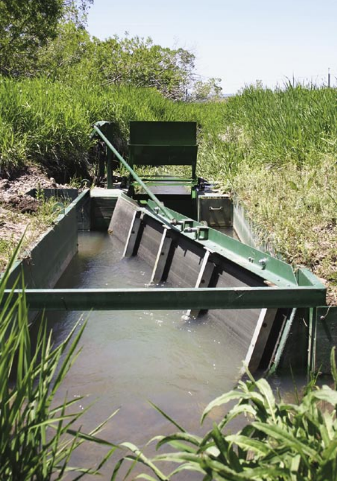
A self-cleaning fish screen at a stream-flow diversion on lower Lassen Creek prevents fish from entering irrigation delivery ditches and becoming stranded.
